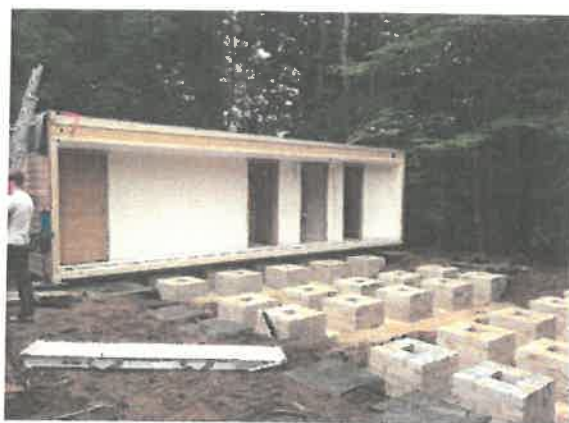
The first piece in place
