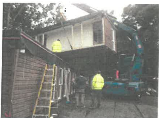
The final piece of the building lowered into place
