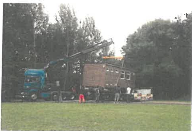
Lowering the first piece of building off the lorry
