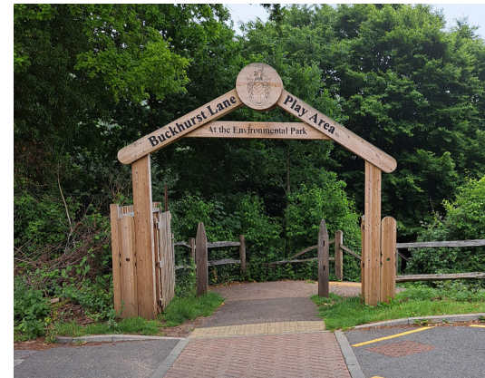
Image 4.11: Current entrance gate to Environmental Park (that leads to Knoles)
