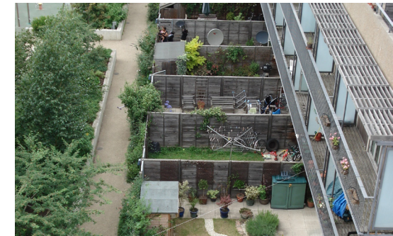
Image 4.16: Pedestrian passageway behind mews housing and gardens
