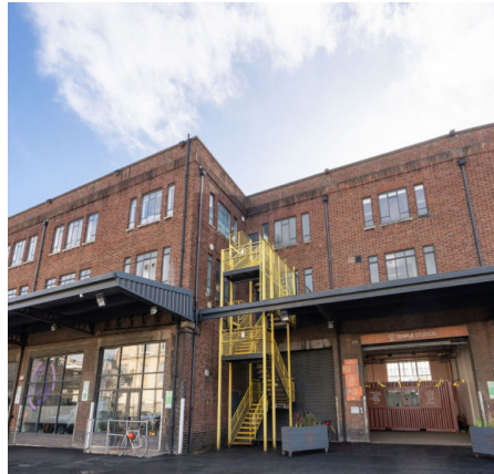
Image 4.9: Workshop units below residential
