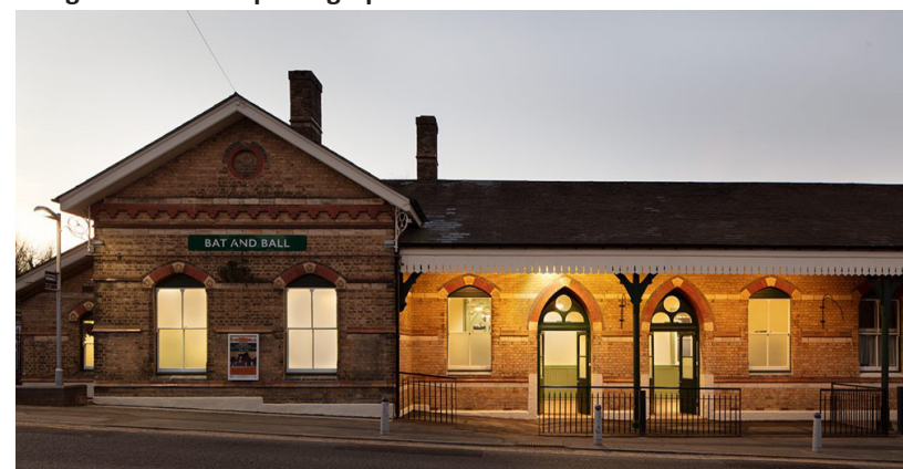
Image 2.3: Recent image of renovated Bat and Ball Station
